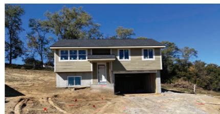
New Construction in Maplewood Circle 120 Maplewood Circle, Glenwood, IA 3 Bed | 1 Bath | $259,000 Jim Hughes 712-520-7300
